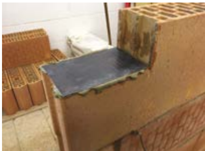
1. A piece of DPC should be laid on the bearings using Zero Plus mortar.
