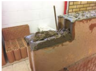
2. The lintels are installed using traditional mortar on the bearings.
