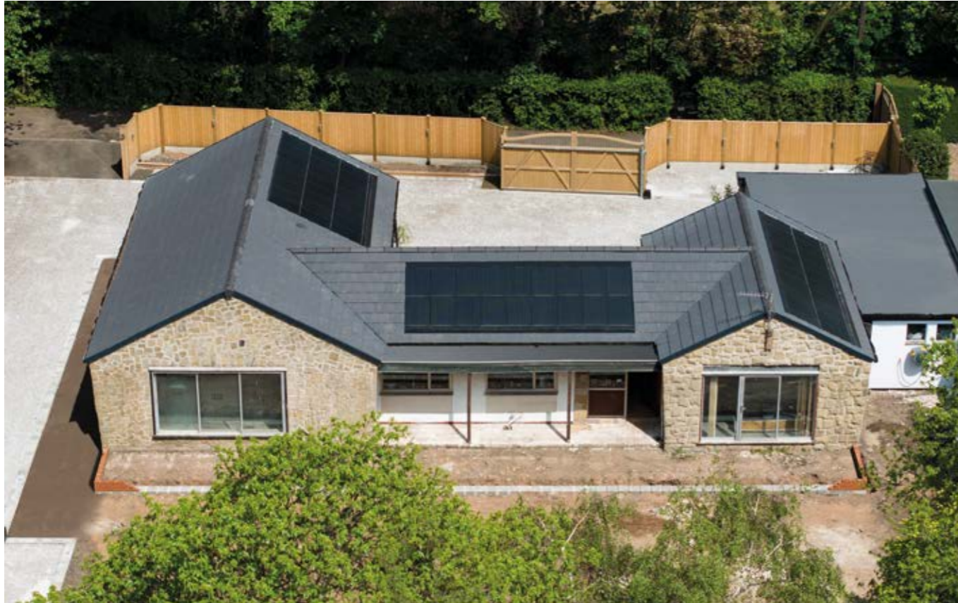
Re-roof (Tiles used - Sandtoft 2020 Antique Slate) - 7.75kWp
