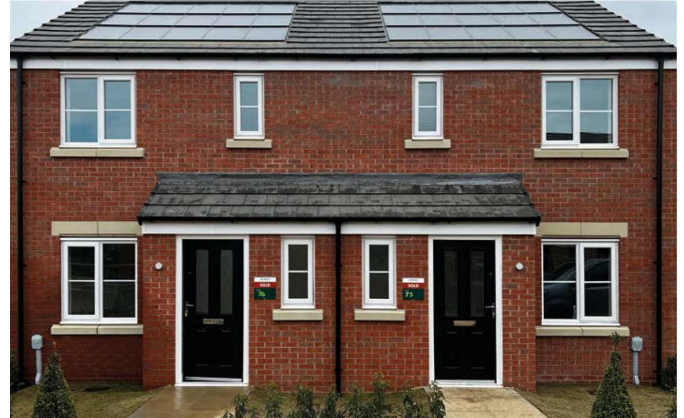
New Build (front and back elevation) - 3.75kWp
