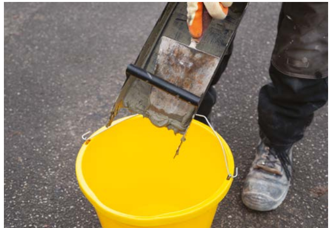
4. Remove any remaining ZeroPlus mortar from the trough before thoroughly washing that out also.
