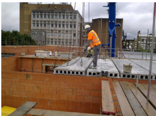
Final positioning utilising lifting eyes.
