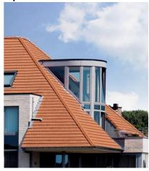
Standard tiles and tile-and-half tiles can be used to finish at the hip. Sandtoft Roll Hip and Multiversal dry hip systems can be used, with Sandtoft clay third round or Duracoat half round or legged angle hip ridges.
