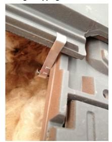
In common with 20/20 tiles, Vauban has a single nail fixing at the head.
