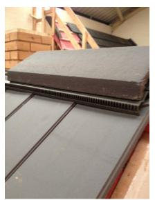
Vauban finishes at the ridge with standard tiles. All Sandtoft dry ridge systems can be used; ie Profile ridge, RollRidge and Multiversal, with Sandtoft clay or Duracoat half round ridge or Duracoat legged angle ridges.
