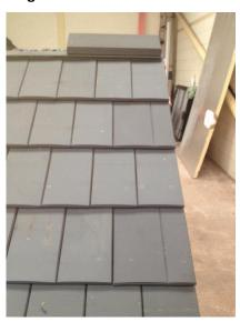
Tiling commences from the right hand verge using standard tiles and RH tile-and-half tiles in alternate courses. Similarly, tiling finishes at the left hand verge using LH verge tiles and LH tile-and-half tiles in alternate courses. The tile-and-half tiles have a mock bond and so look in keeping with the general tiling.
