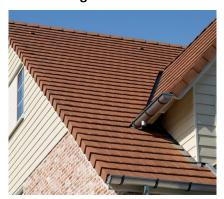
Purpose made cloak verge tiles are available for Vauban. These are in tile and tile-and-half width cloaks, for use in alternate courses at left and right hand verges.
