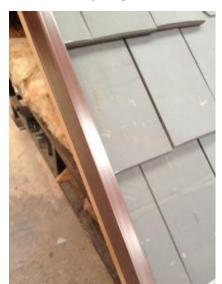
The 20/20 MF dry verge will not fit Vauban and the gauge is too small for LF dry verge or Multiverge.
