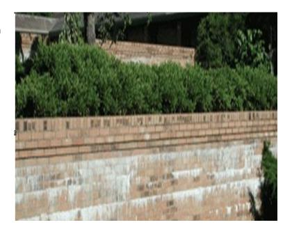
Although white in appearance, the staining is distinctly different to the soluble salt deposits (efflorescence) which can sometimes appear on brickwork. The initial staining can be removed with water and brushing before it carbonates, but once reaction has taken place an acid solution will be necessary to break down the material.
