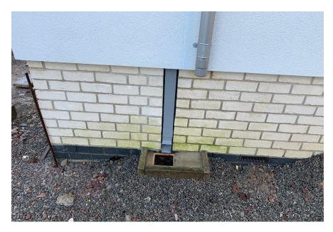
Surfaces that are exposed to driving rain or with design features which result in poor shedding of water are at particular risk. Mosses tend to be found on surfaces where soil and dirt has accumulated.
